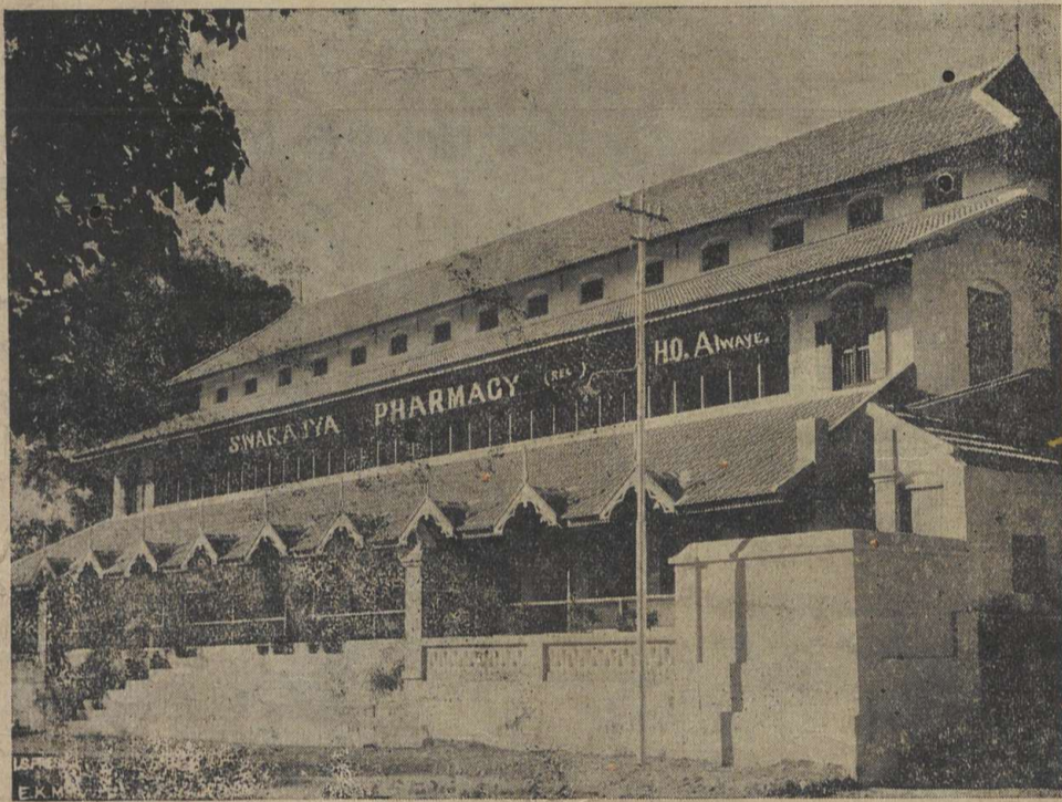
Front view of the newly constructed 'SWARAJYA PHARMACY' building
