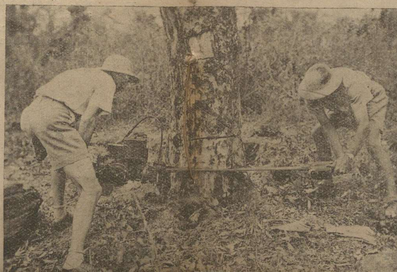
(Below) Here are two men using an electric saw which can cut even the largest of trees in the space of a few minutes.
