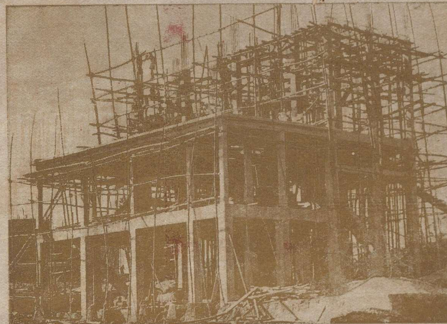
A view of the Plant from the river side. Concreting is in progress for the columns above the first floor. Photo taken on 23rd Nov. 1953
