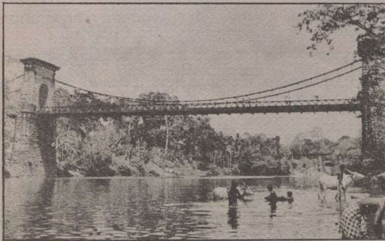
The suspension bridge at Punalur, across the Kallada river. This bridge is now of archaeological interest;- a souvenir of British engineering of yore.
