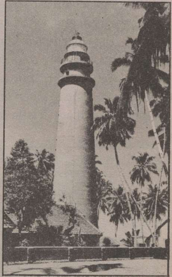
A silent sentinel since the turn of the century;- the Thangassery light house
