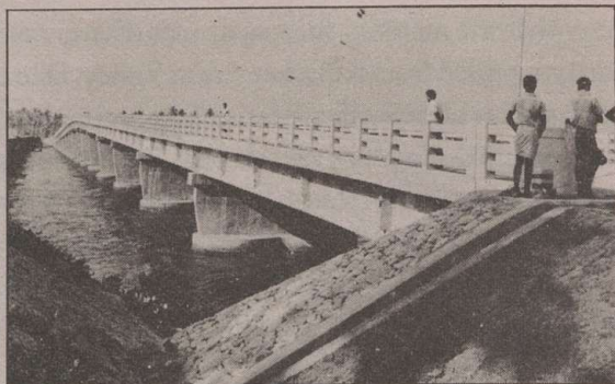
The Neendakara bridge over the Ashtamudi Lake on N.H. 47
