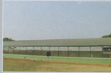
KCA CRICKET STADIUM PERINTHALMANNA, INDOOR FACILITIES
